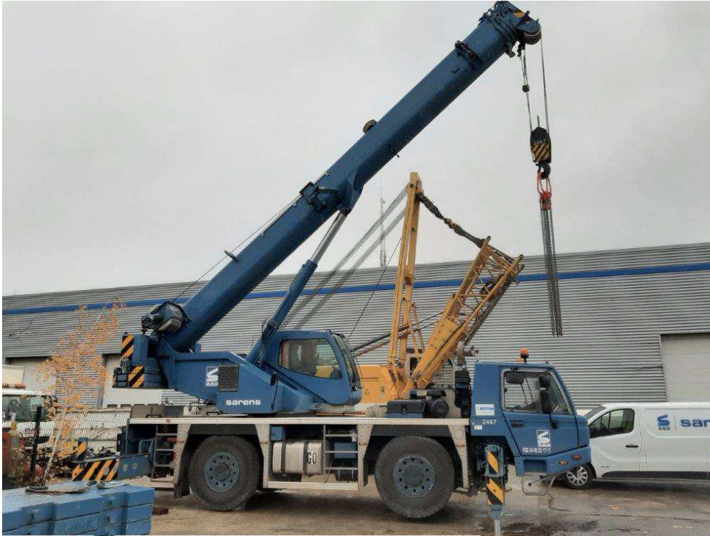
Equipment: FAUN ATF 40G-2 (2467) LOCATION: FRANCE – PARIS
