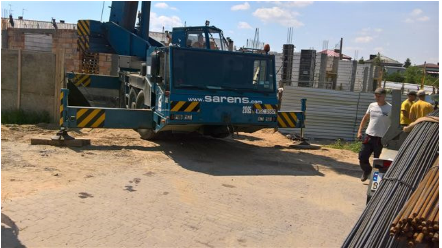
Equipment: Terex-Demag AC50 (2095) LOCATION: Poland
