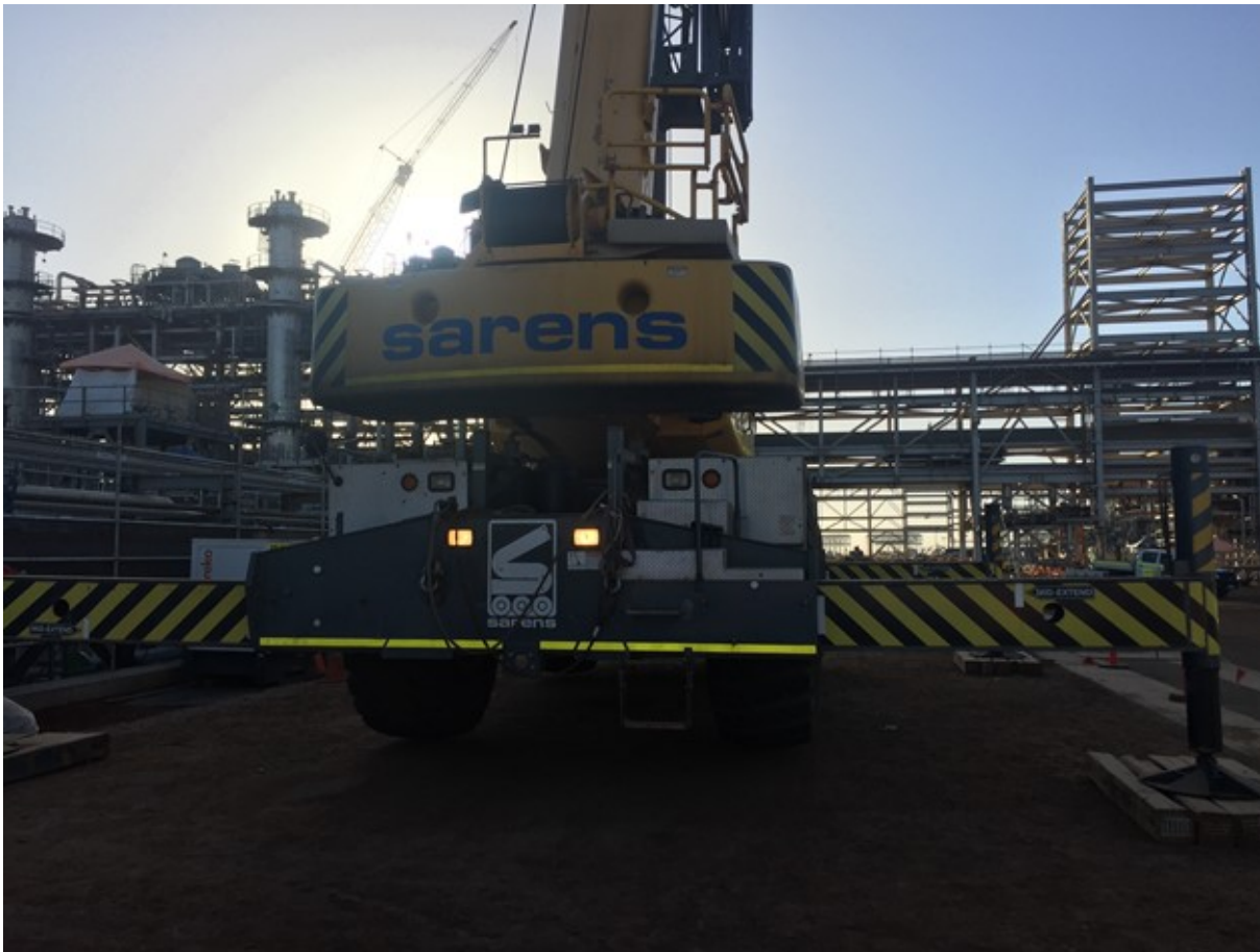
Equipment: GROVE RT 9150 (4559) LOCATION: Australia
