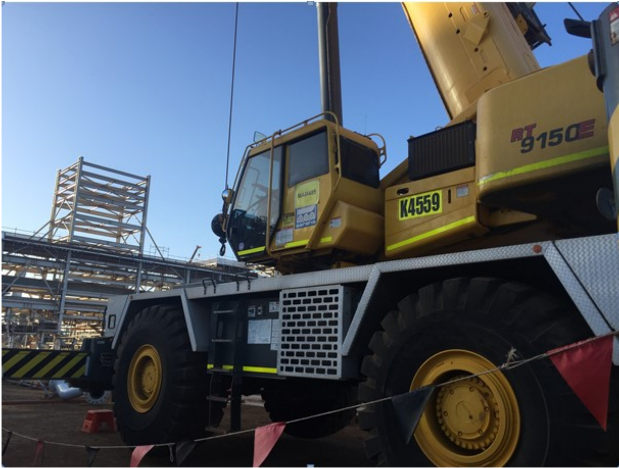
Equipment: GROVE RT 9150 (4559) LOCATION: Australia
