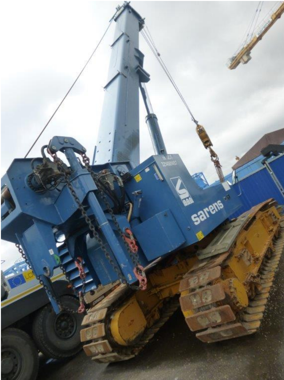
Equipment: Sennebogen 683 R-HD (2629) LOCATION: Poland
