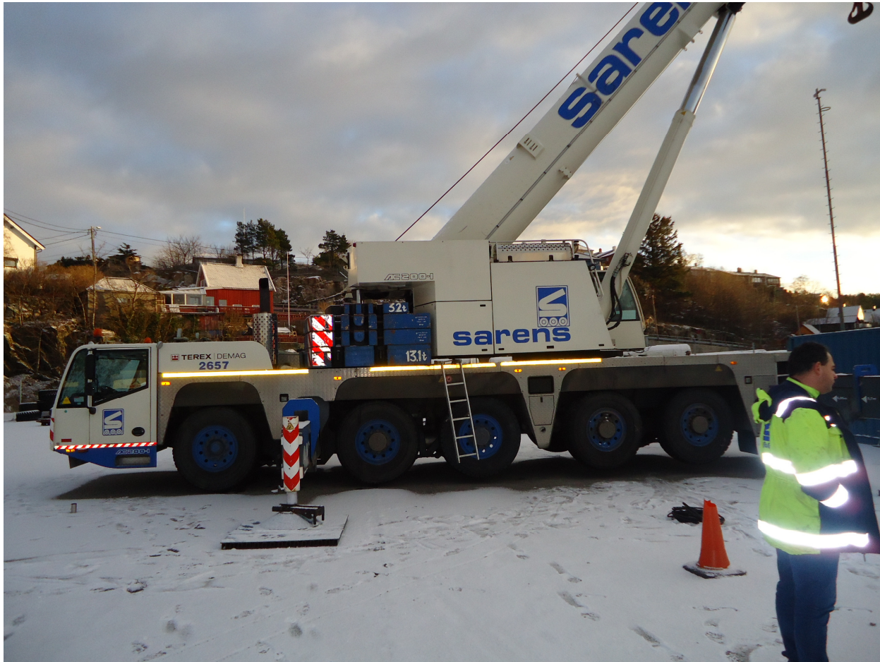
Equipment: Terex-Demag AC 200-1 (2657) LOCATION: Europe
